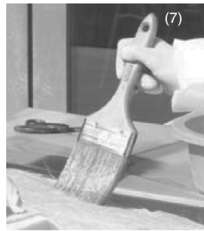
The epoxy thermosetting resin is layed up
