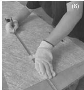
The glass fiber is cut
